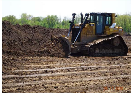
Stripping topsoil at onset of construction
