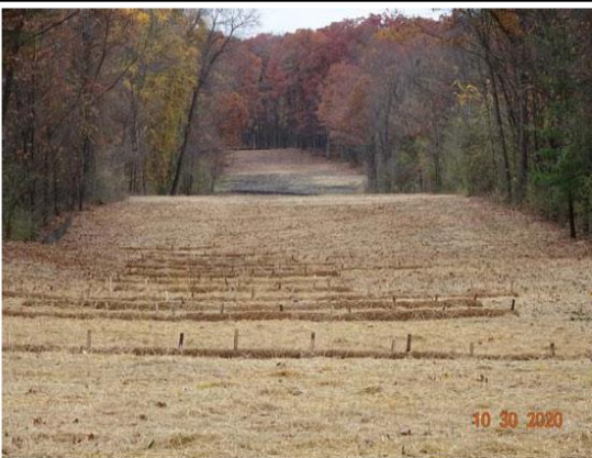
Crimped mulch, plus biologs on potentially erosive slope
