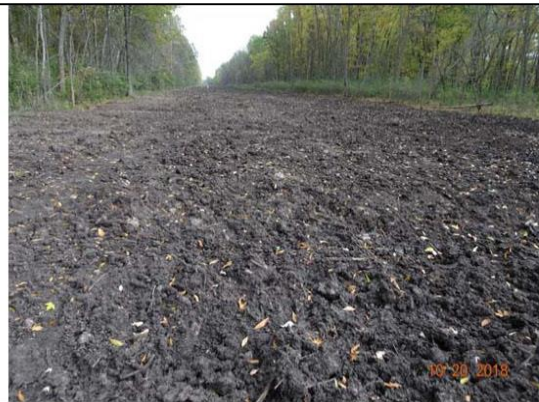
Topsoil restored after pipeline installation
