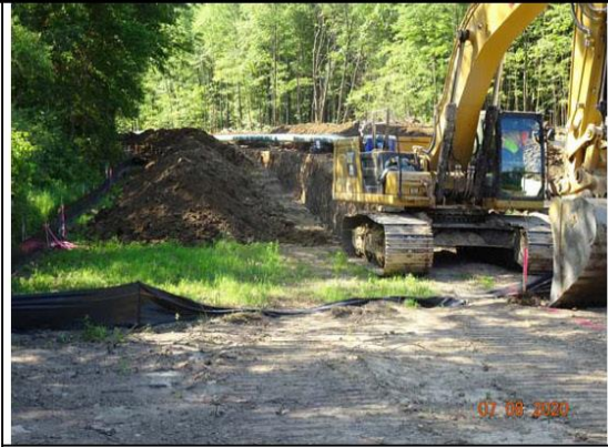
Stripped topsoil – left side of photo
