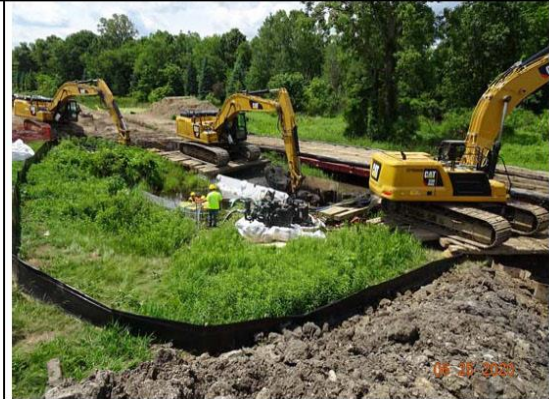
During pipeline installation, with dam & pump stream-flow bypass
