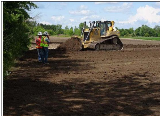
Restoring topsoil
