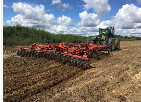
Decompacting subsoil during restoration
