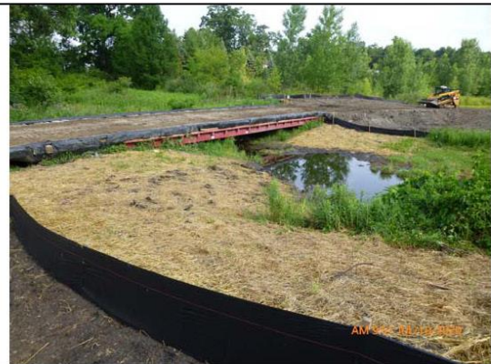
After pipeline installation – banks restored except bridge location
