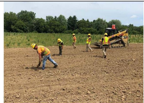
Removing excess rock
